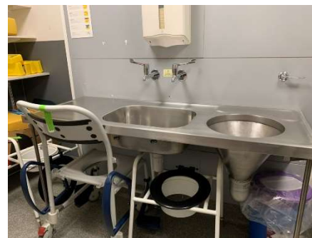
Figure 1a Dirty utility above left: with no set-down space by the macerator and insufficient space for waste disposal.
